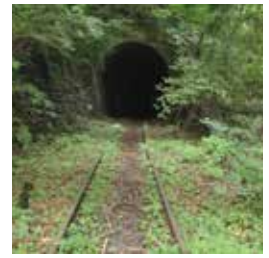
Unused Tunnel. Photo from Wikipedia.
